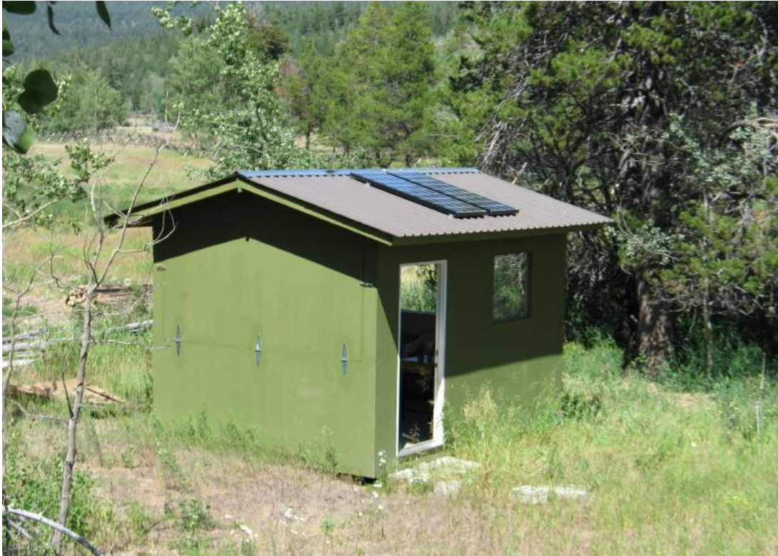
Figure 5. Banding station showing solar panels on roof.
