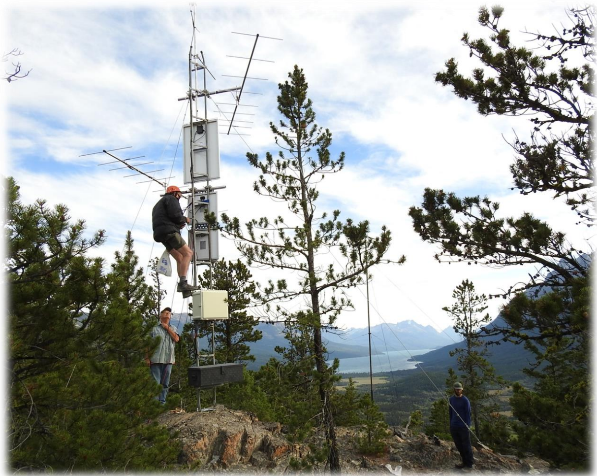
Setting up the Motus receiving station, the two 9-element antennas and top solar panel are part of the Motus setup
